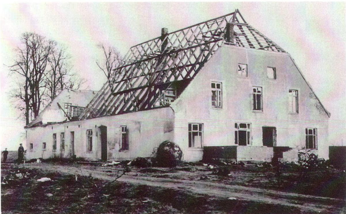
Abriss Hof Rose, 1964
